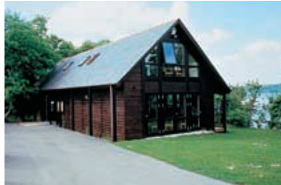
A sailing clubhouse where the scale has been reduced by utilising the roof space for some social and office accommodation and by treating the cladding and joinery in a stain of uniform colour.
